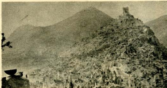
Not a building remained intact.
